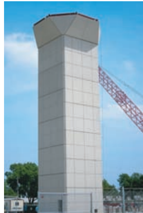
The new Air Traffic Control tower under construction at Wittman Regional Airport, Oshkosh, Wis. When completed, controllers will have a birdseye view of all runways at their perch 120 feet above the ground. In comparison, the old tower is only 67 feet AGL.
