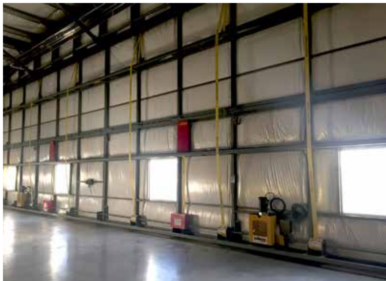
The Life Flight liftstrap door is well insulated. Inside the hangar are 24/7 crew quarters for flight crews and administrative staff.
