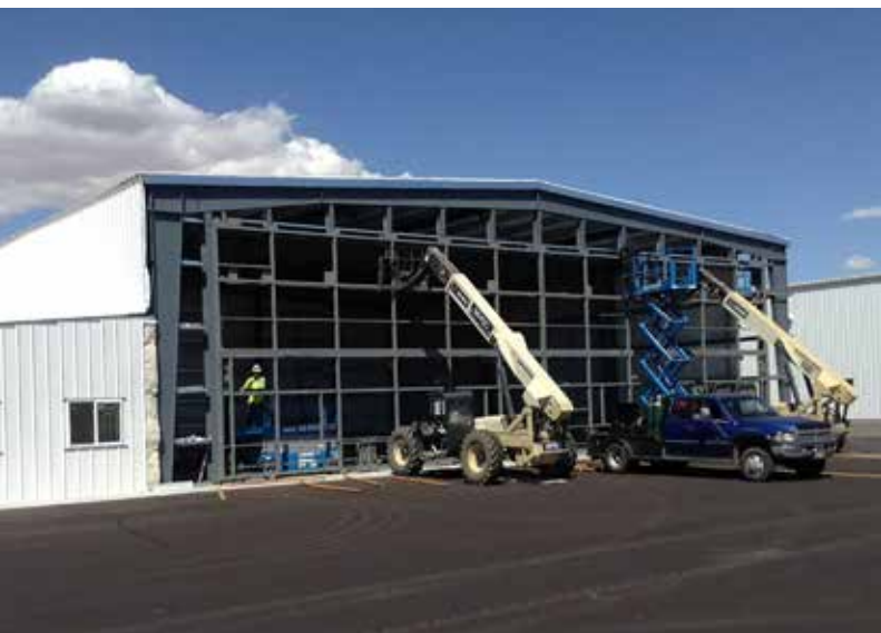
The Schweiss bifold 70-foot by 17-foot liftstrap door is equipped with autolatches and is wind-rated at 120 mph.
