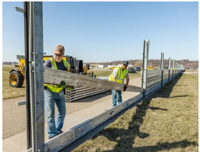
A MAC crew installs a section of the temporary flood wall at St. Paul Downtown Airport on April 13, 2023.
