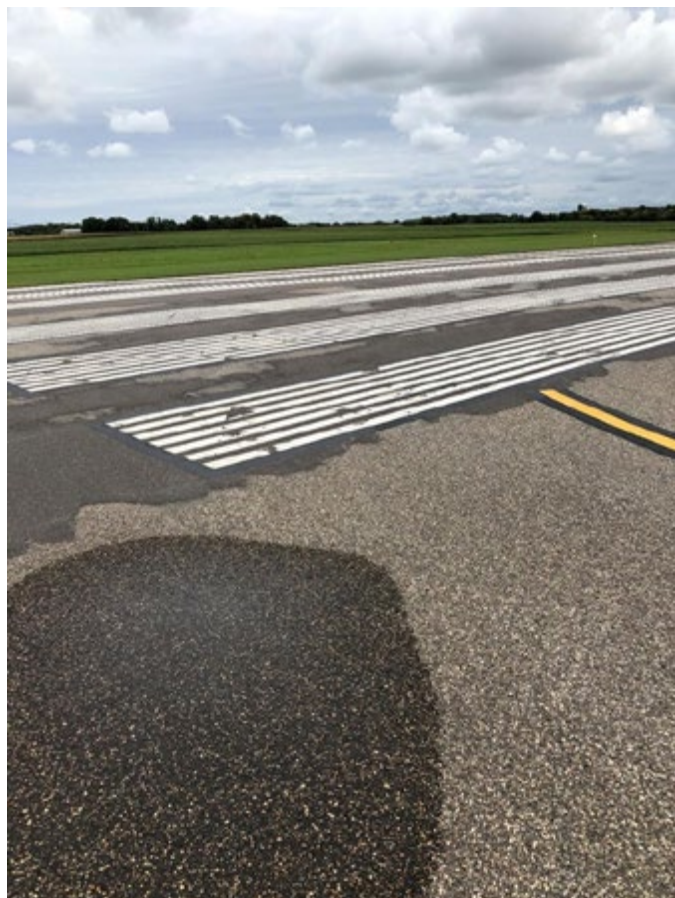
Example of threshold at the end of its useful life
